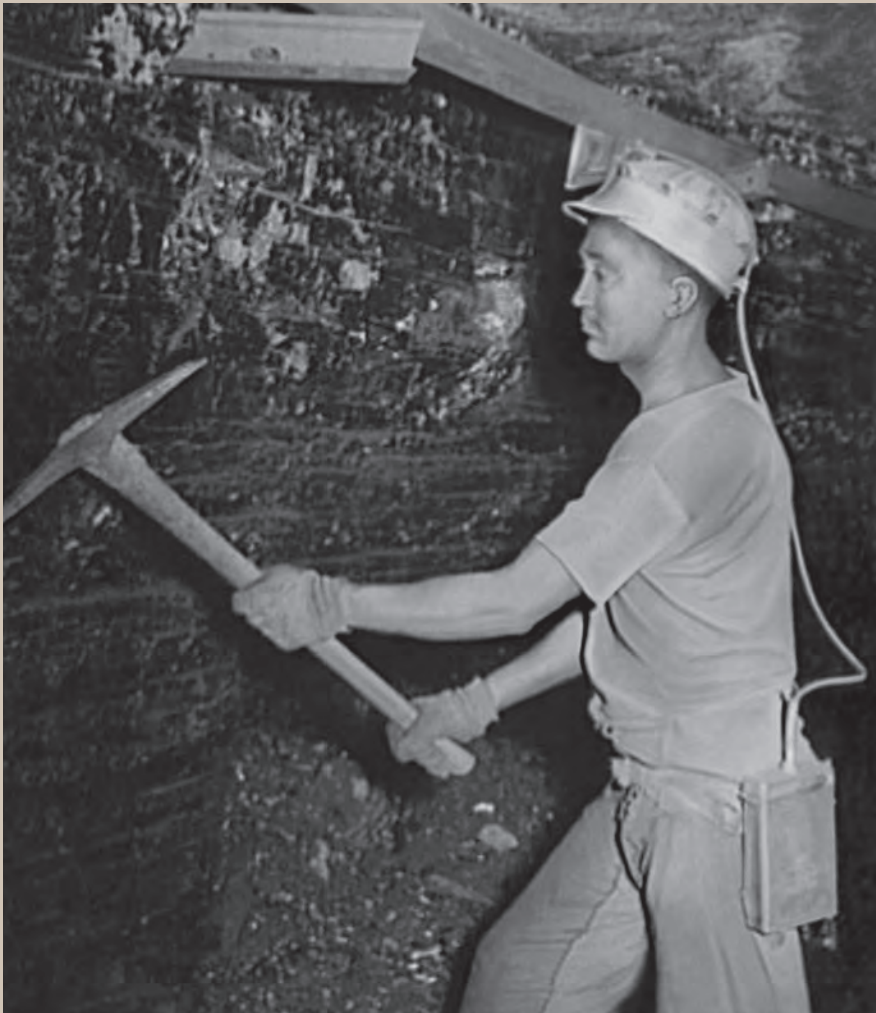
One of the basic tools in early mining was the pick axe, which was used to break the coal loose from the veins. Old Ben #8, West Frankfort.
