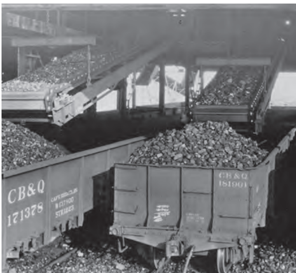
Top: Picking tables where workers removed roof shale from lump coal before loading into rail cars. ISGS, circa 1920. Chicago, Wilmington & Franklin Coal Company, Orient No. 2 Mine, Franklin County.
