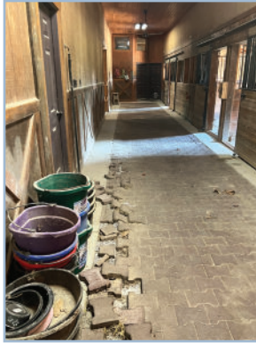
The tour included a view of damage to the floors and ceiling of the horse barn, and misalignment of garage doors. All were grateful to the property owners for providing the opportunity to see mine subsidence damage first-hand.
