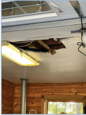
The tour included a view of damage to the floors and ceiling of the horse barn, and misalignment of garage doors. All were grateful to the property owners for providing the opportunity to see mine subsidence damage first-hand.
